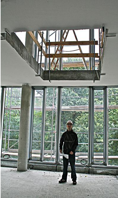
Figure 12: The construction site earlier this year.
